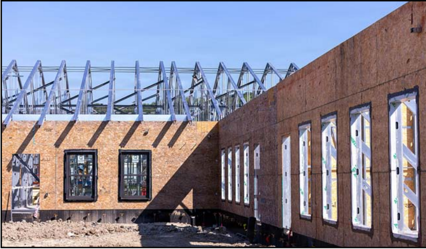
Photos by Christine Reinhardt/U.S. Army Corps of Engineers, Kansas City District
